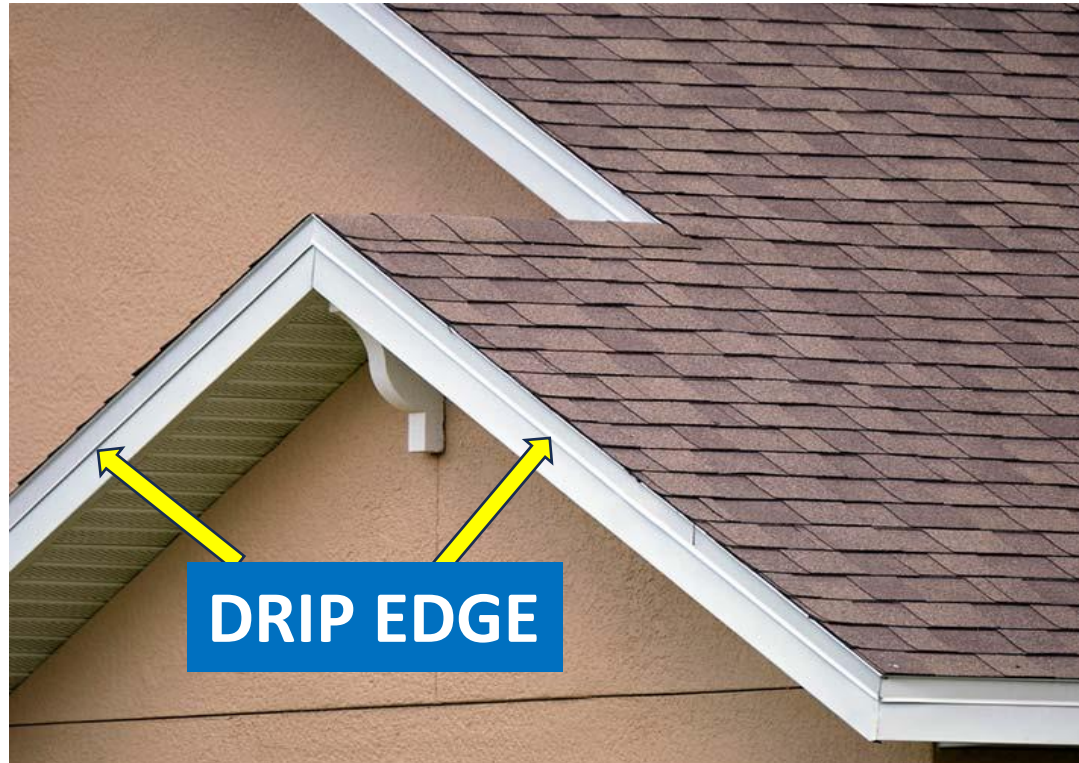
Drip Edge Moldings on Full Length of Roof “Rakes” (Peaks)
